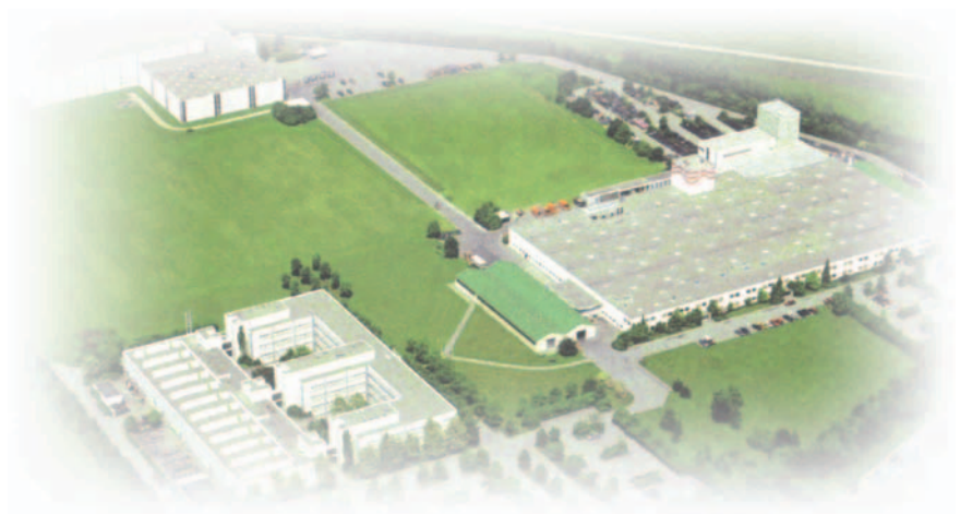
Energy Division Headquarters Ottobrunn, Munich/Alemania
